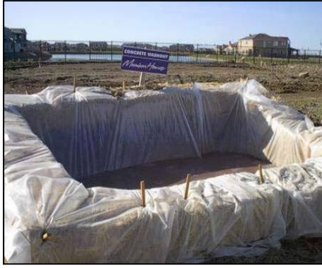
Plate 3.1 Concrete washout area
