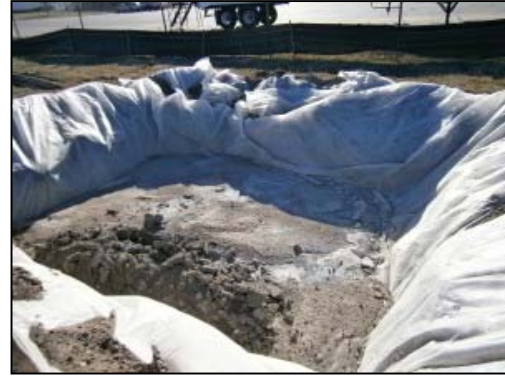
Plate 3.2 Concrete washout area
